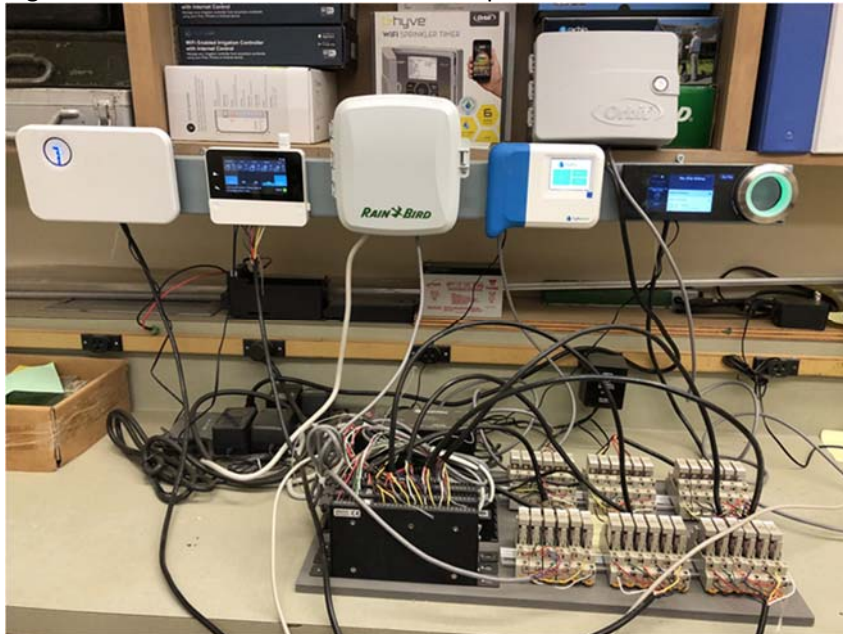
Figure 1. Controller installation and Setup in the Lab
