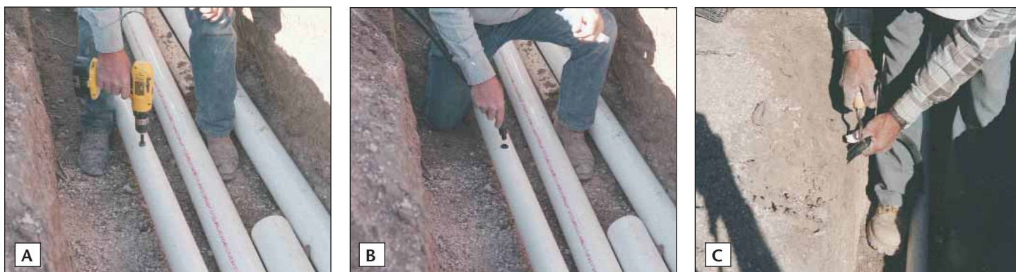
Figure 9. Drilling the manifold (A), inserting the grommet and the PVC hose (B), and connecting the PVC hose to the drip tape (C).
