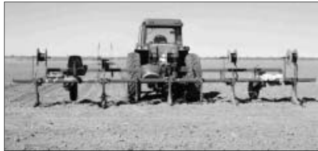
Figure 12. Installation of a subsurface drip irrigation system.
