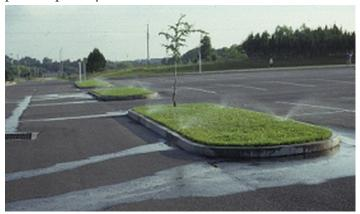
Figure 2. Make sure that irrigation systems are applying water to grass, not pavement. Credits: Michael Dukes
