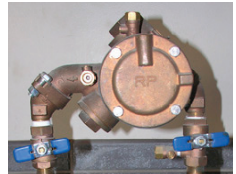
Figure 4: Reduced Pressure Device.
