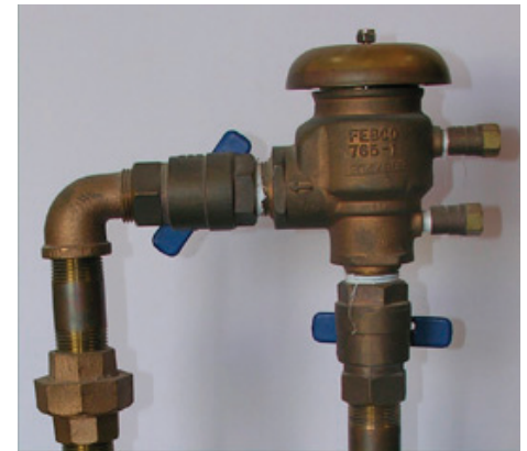
Figure 3: Pressure Vacuum Breaker.
