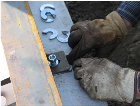
Figure 5b. The I-beam base of the rail system is bolted into the concrete tracks with slotted brackets to allow for expansion and contraction.
