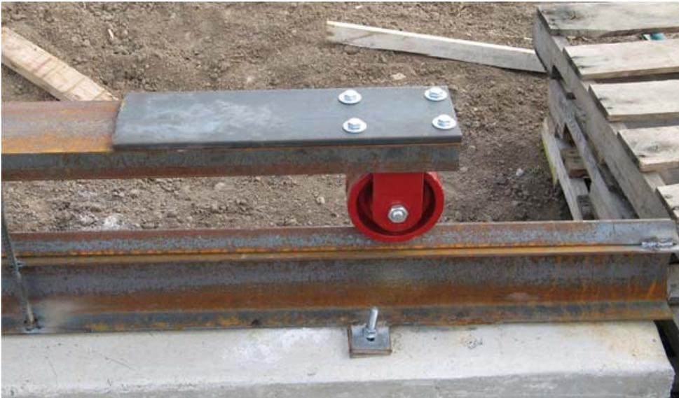
Figure 6. Angle iron forms the top of the rail system and is welded onto the I-beams. Also shown is the C-channel that forms the base of the roof structure to which the wheels are attached.
