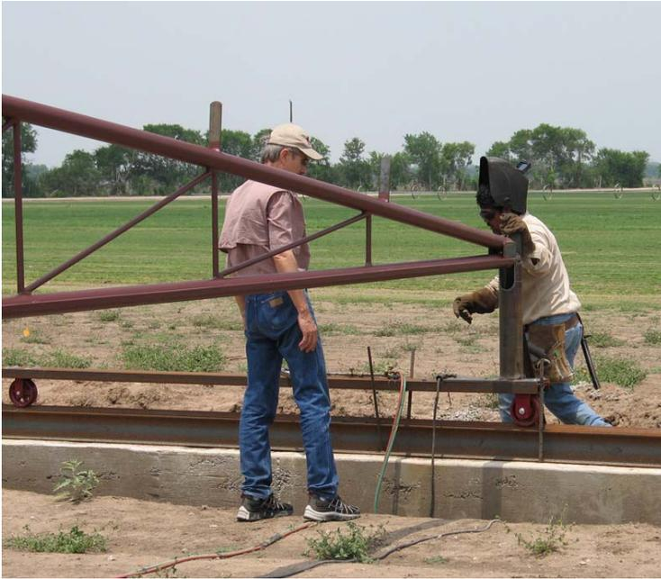
Figure 7. The roof is elevated to provide 4 foot of ground clearance using pipe welded to the c-channel forming the base of the roof structure.
