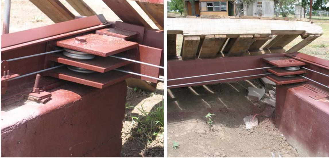
Figure A-3. Corner Pulley
