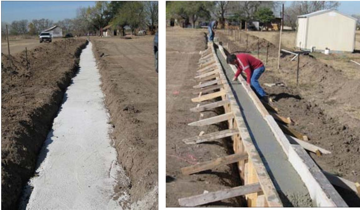
Figure 4. Construction of the track system composed of a footing and a concrete slab.
