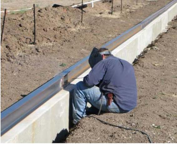
Figure 5a. The base of the rail system is composed of I-beams welded together.
